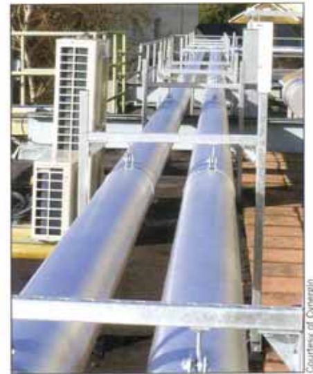
From the Women's Health & Maternity Unit boiler room, the low temperature hot water will be taken via a twin-run of 220 metre stainless steel pipework across the roof at the back of the adjacent tower block, and then down to its second floor, into the so-called 'ZPL8' main tower plant room.
