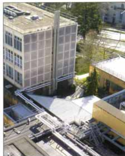
From the Women's Health & Maternity Unit boiler room, the low temperature hot water will be taken via a twin-run of 220 metre stainless steel pipework across the roof at the back of the adjacent tower block, and then down to its second floor, into the so-called 'ZPL8' main tower plant room.
