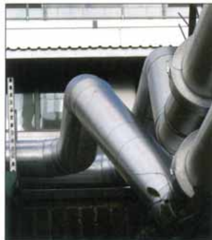
The Women's Health & Maternity Unit at the YDH site. Centre: The new flues at the side of the unit. Right: Low temperature hot water ring pipework leaving the Women's Health & Maternity Unit plant room on its way to the main hospital's plant room.
