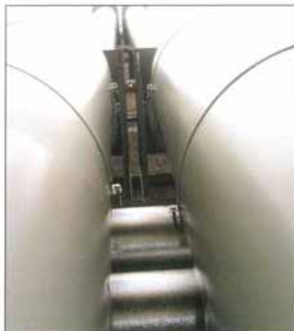
The Women's Health & Maternity Unit at the YDH site. Centre: The new flues at the side of the unit. Right: Low temperature hot water ring pipework leaving the Women's Health & Maternity Unit plant room on its way to the main hospital's plant room.
