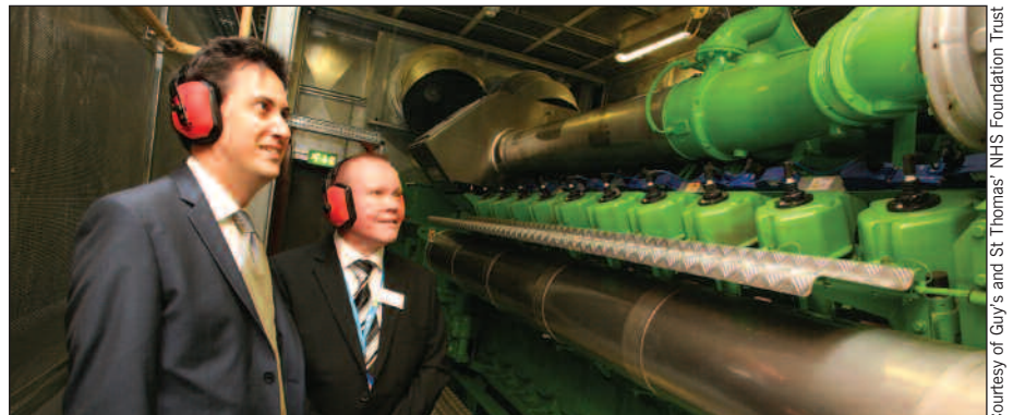
Ed Milliband, at the time Secretary of State for Energy and Climate Change, visits St Thomas' Hospital in September 2009 to officially 'open' the new Jenbacher CHP plant there. He is pictured with David Porter, head of engineering at Guy's and St Thomas' NHS Foundation Trust.
