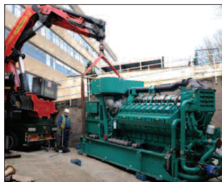
The existing boiler at the Royal Berkshire Hospital, Reading, being removed, prior to Dalkia's installation of equipment including a new Cogenco 2 MWe CHP unit, incorporating a Cummins engine (centre), and a 1 MW Danstoker waste heat boiler (right).
