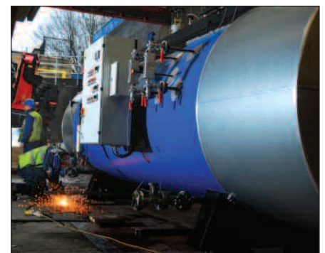
The existing boiler at the Royal Berkshire Hospital, Reading, being removed, prior to Dalkia's installation of equipment including a new Cogenco 2 MWe CHP unit, incorporating a Cummins engine (centre), and a 1 MW Danstoker waste heat boiler (right).
