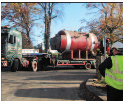
The existing boiler at the Royal Berkshire Hospital, Reading, being removed, prior to Dalkia's installation of equipment including a new Cogenco 2 MWe CHP unit, incorporating a Cummins engine (centre), and a 1 MW Danstoker waste heat boiler (right).
